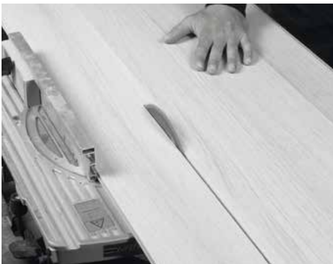
Last or first panel: saw to size.
