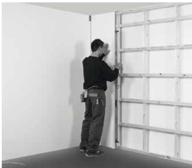
Place the first panel level.
