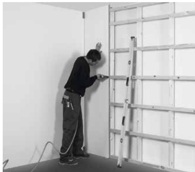
Attach into the notches of the Uniclic® profile (every 400mm).
