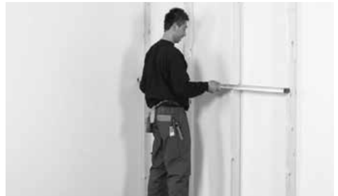
Always ensure that the substructure is fitted vertically.
