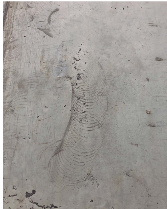
Mark left in the concrete by the vibrator.
