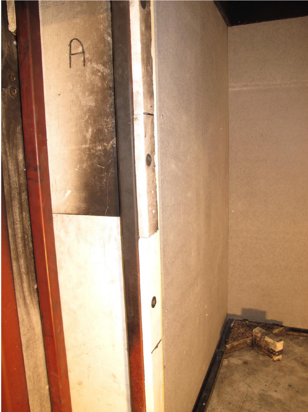
Photo no 2 Prior to test "Fibersementplate BF"
