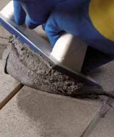
Spreading Kerapoxy CQ using a MAPEI float
