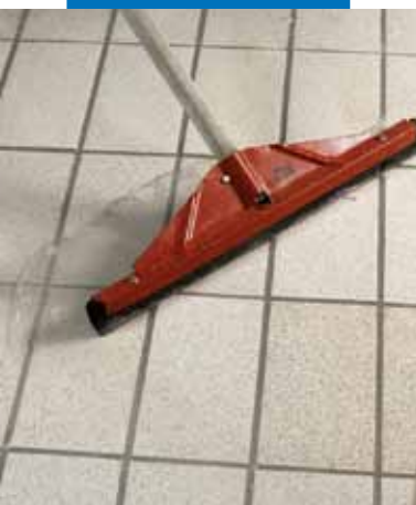
Removing excess liquid using a rubber squeegee
