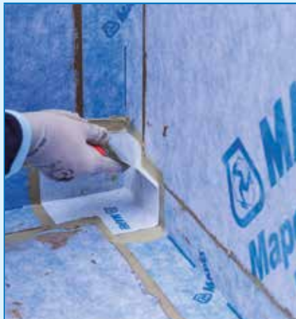
Application of MAPEGUARD IC in the internal corner with MAPEGUARD WP ADHESIVE
