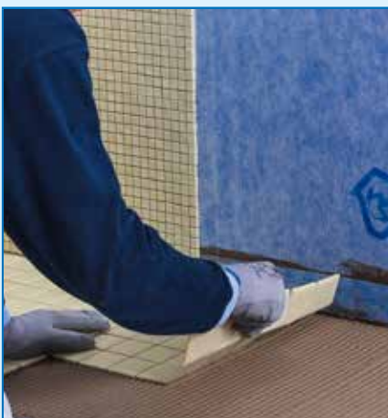
Tile installation with a cementitious tile adhesive
