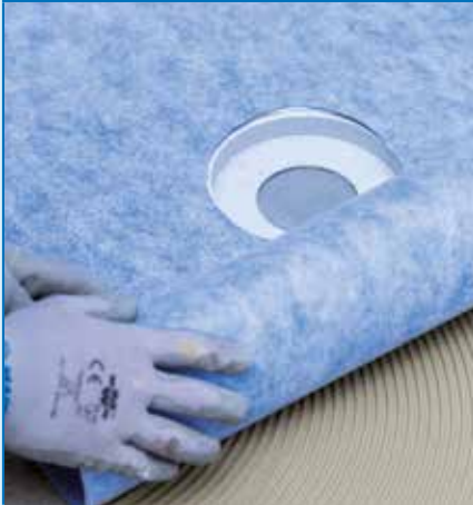
Unrolling MAPEGUARD WP 200
