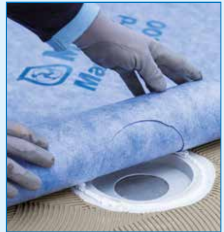
Laying of MAPEGUARD WP 200
