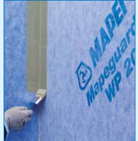
Application of MAPEGUARD WP ADHESIVE before MAPEGUARD ST to seal the junction between two adjoining sheets
