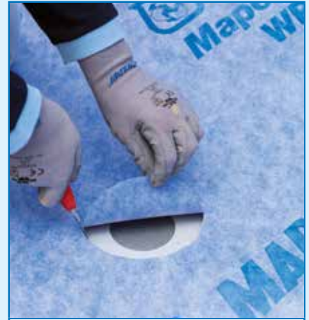
Cutting the membrane
