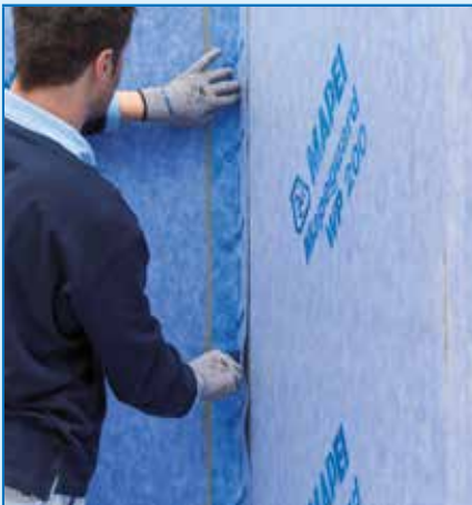
Application of MAPEGUARD ST onto MAPEGUARD WP ADHESIVE
