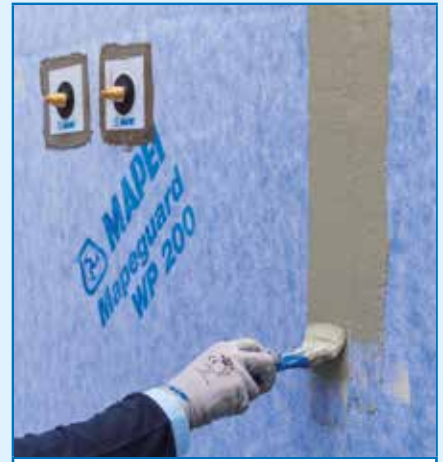
Application of MAPEGUARD WP ADHESIVE before MAPEGUARD ST to seal the junctions between two adjoining sheets
