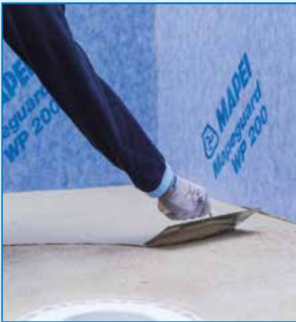
Application of the cementitious tile adhesive
