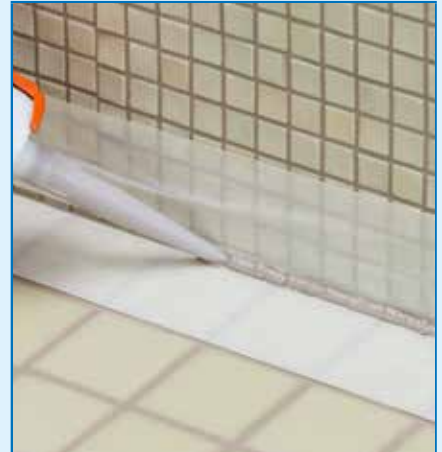
Application of the sealant in all corners
