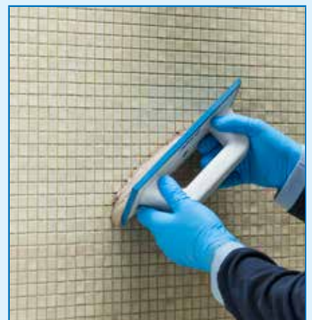
Grouting of the joints
