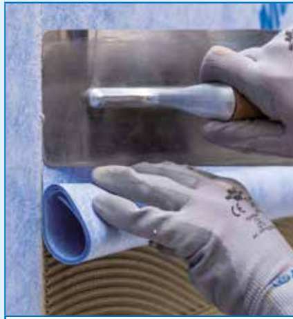
Application of the second sheet of MAPEGUARD WP 200
