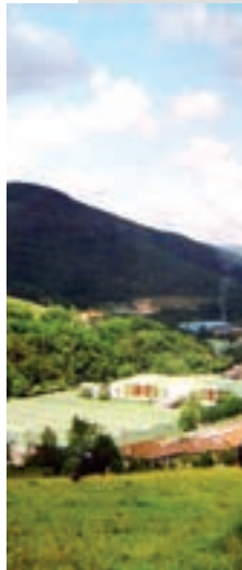
Gerflor Tarare manufacturing plant
