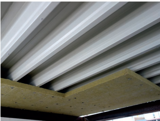
Figure 9. System ISOVER FireProtect® for fire protection of corrugated steel is characterized by light weight and small height, but also a direct fixing to the corrugated steel without need of help of suspension construction
