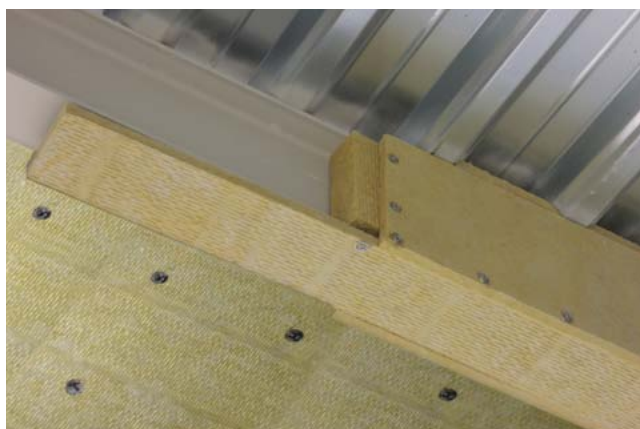
Fig. 1 - Example of use ISOVER FireProtect® 150 (ISOVER Tank Roof Slab 20 kPa)
