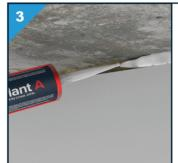
Apply Multisealant A generously to the joint to prevent air bubbles.
