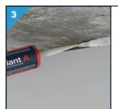
Apply Multisealant A generously to the joint to prevent air bubbles.
