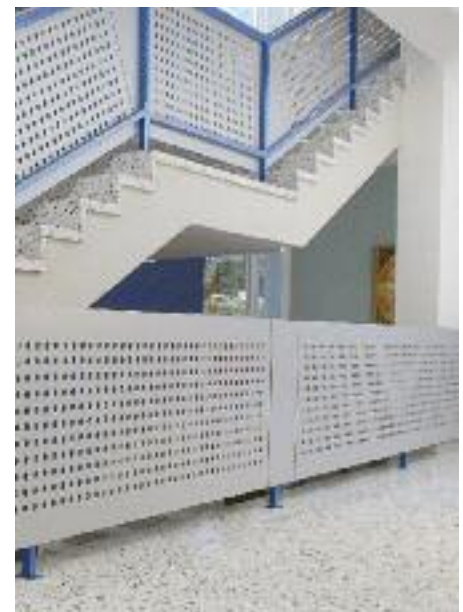
STAIRCASE RAILING WITH HOLES
