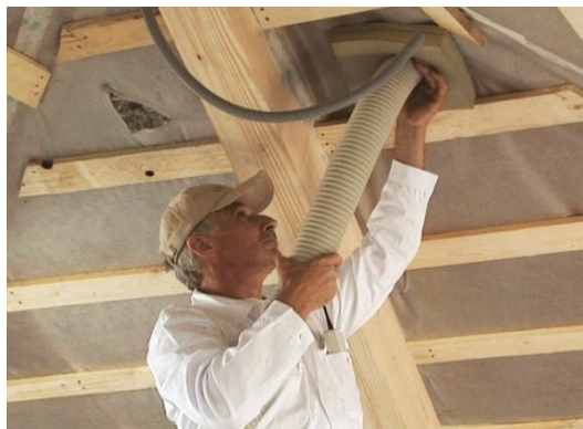
Figure 4: Cellulose insulation in a pitched roof (a: left side and b: right side)
