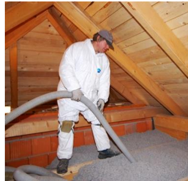
Figure 3: Cellulose insulation in open attics
