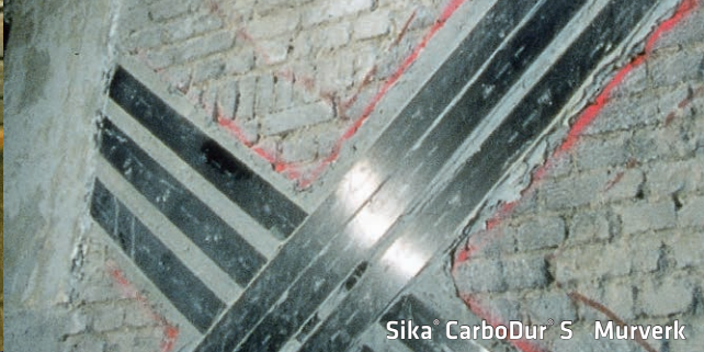
Sika CarboDur S Forsterket betongdekke
