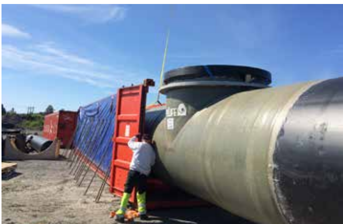
Picture 7 - OD2000 mm T-piece with reinforcement
