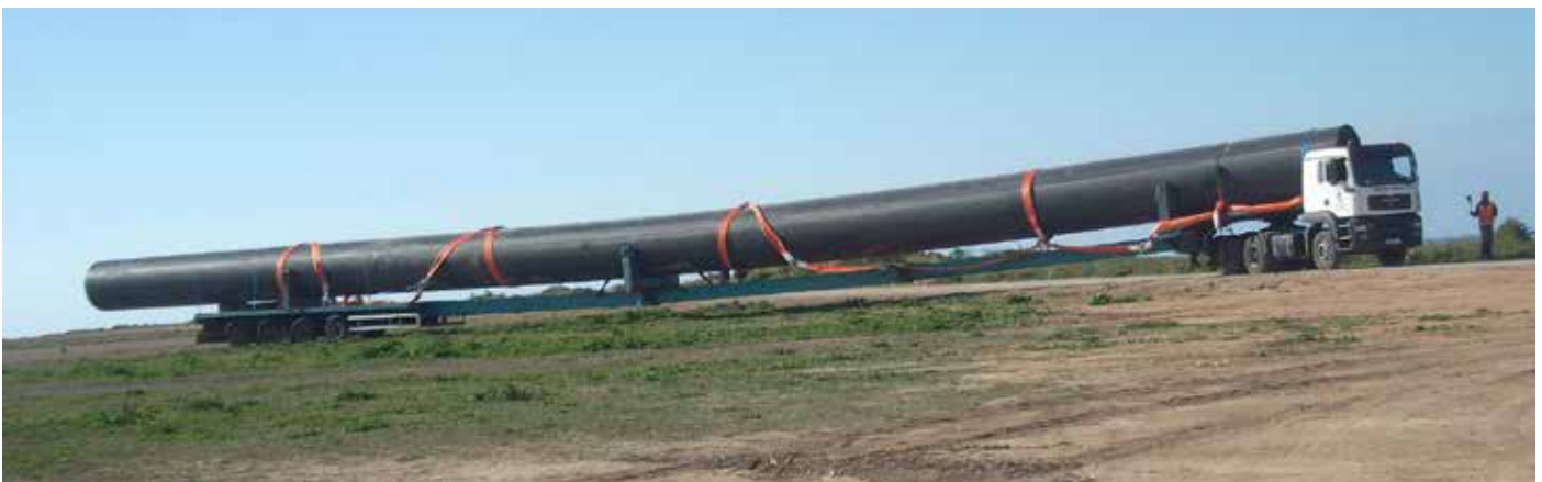
Picture 11 - Innovative on site transport of OD2100 mm in Morocco
