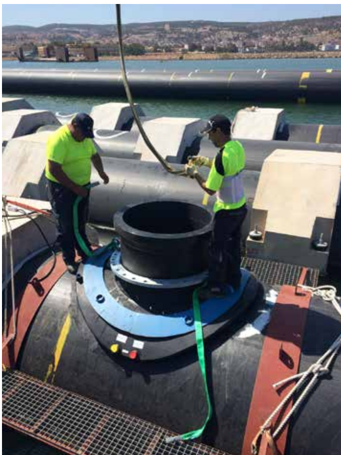
Picture 4 - Preparing the saddle for welding on site
