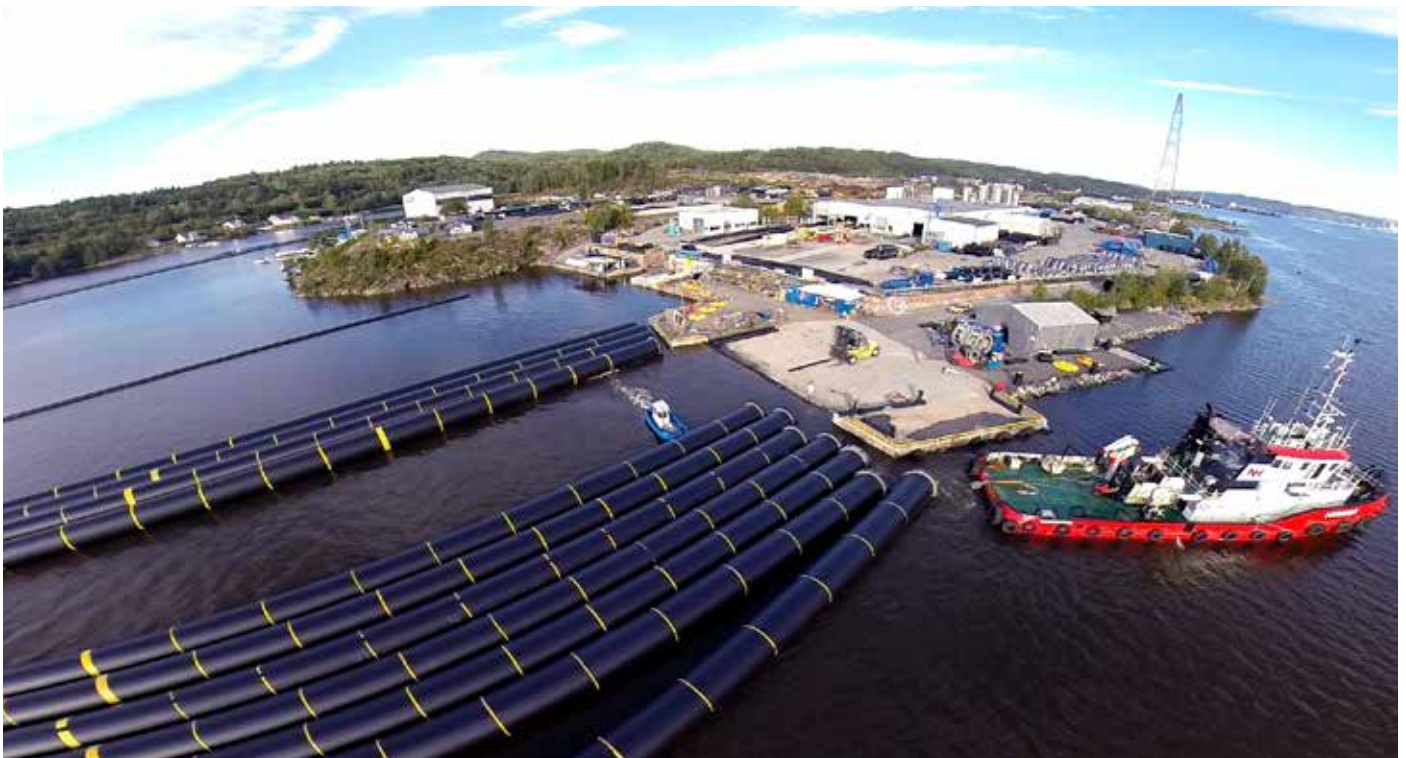
Picture 1 - Pipelife Norge Stathelle plant
