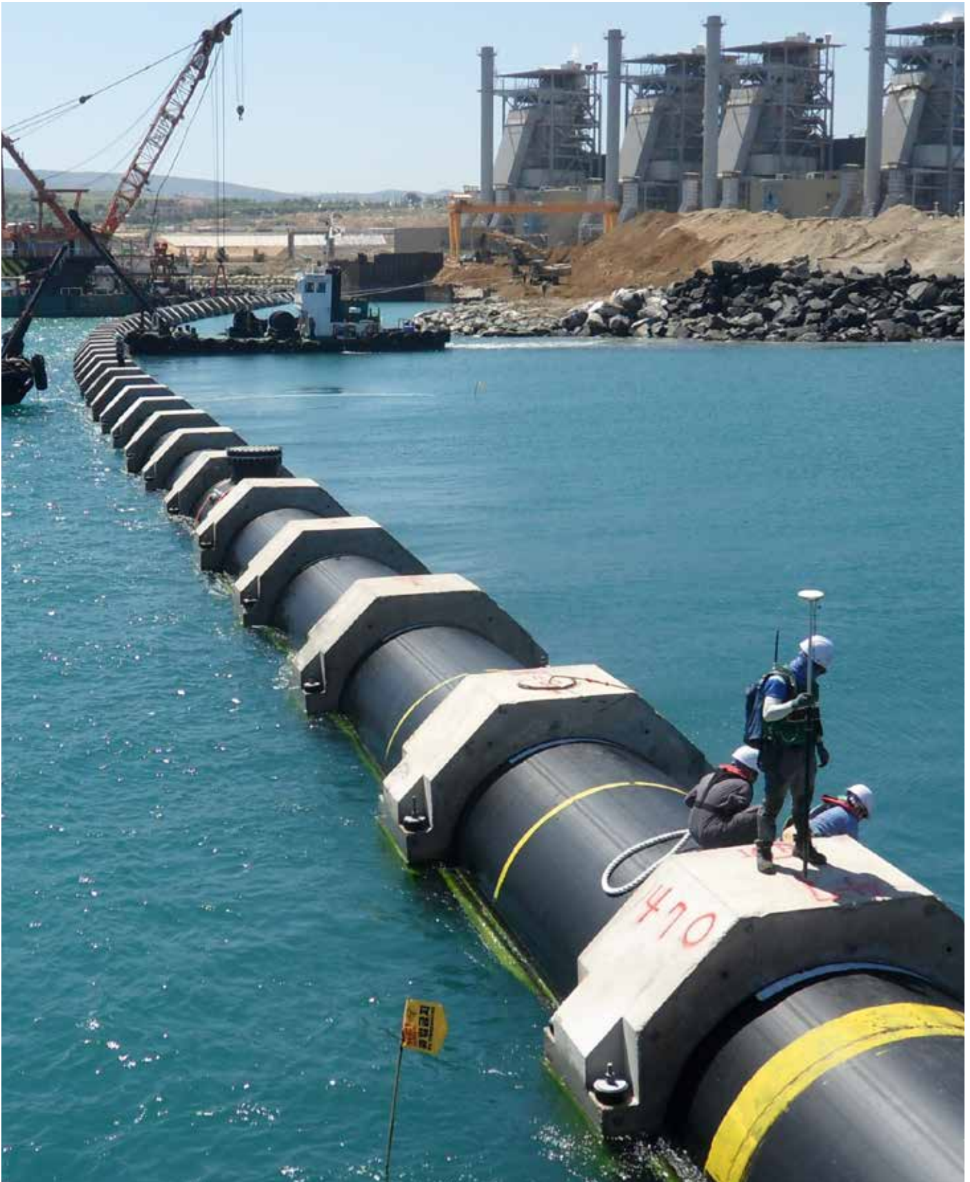
Picture 10 - Beginning of submerging of OD2500 mm SDR26 pipe
