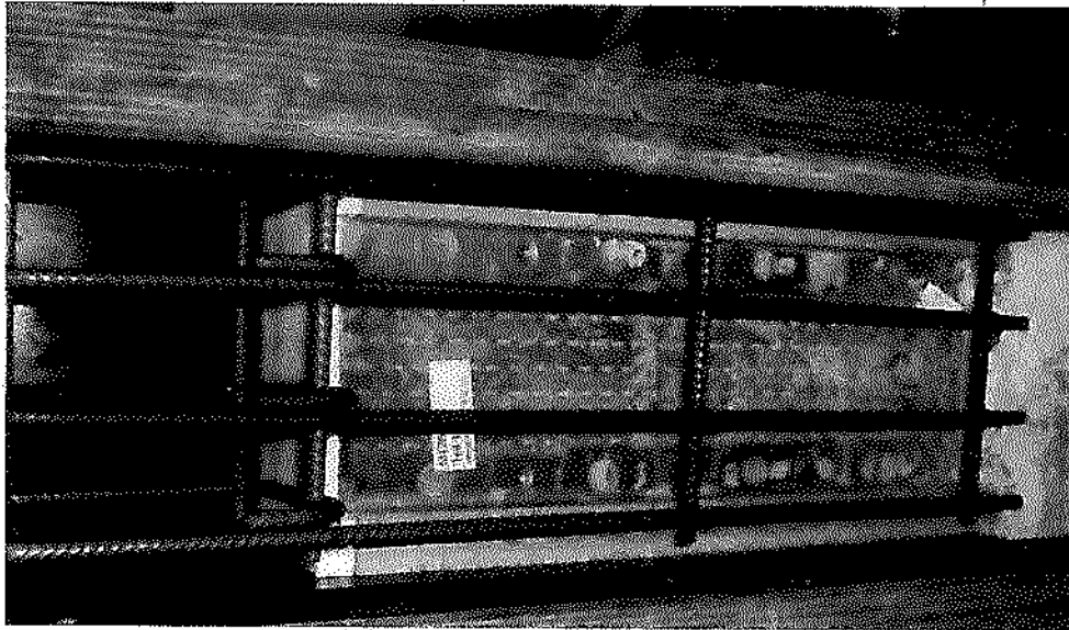
Fig. B7: Shear test in longitudinal direction with reinforcement continuity system: Test specimen prior to the concreting of the second part
