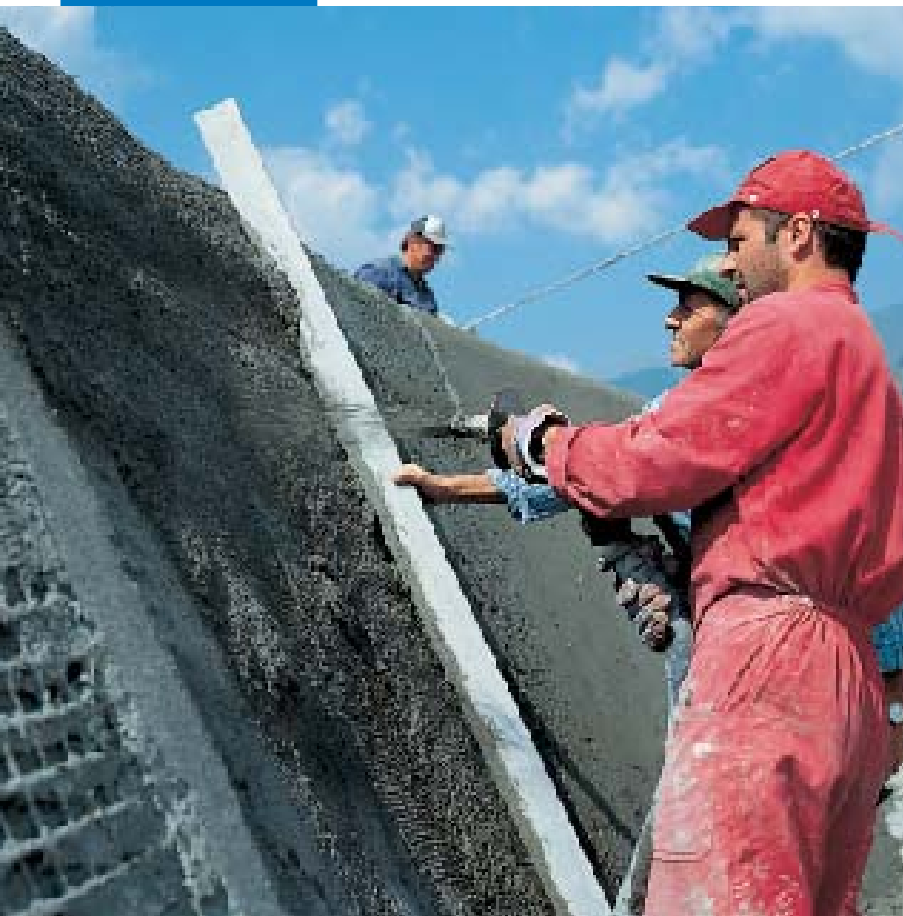
Spray application of Mapegrout T40
