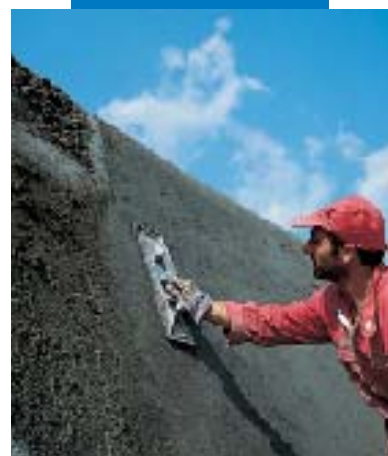
Finishing of Mapegrout T40 with darby
