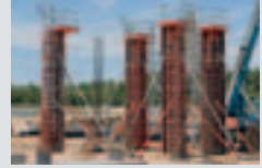
Column Formwork
