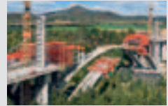
Bridge Formwork
