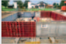
Wall Formwork
